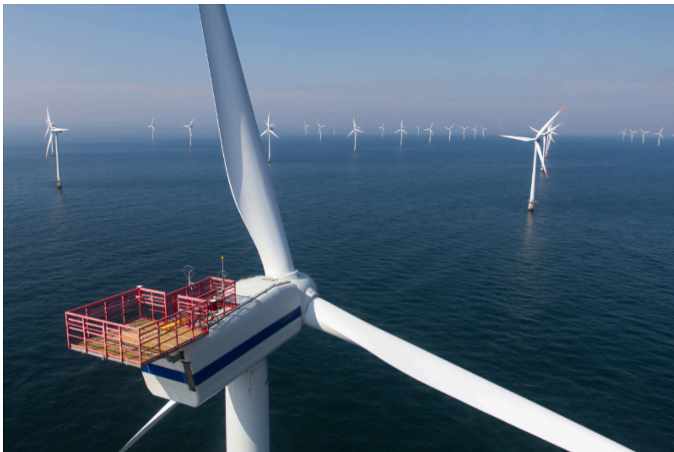
Offshore Windparks. Foto: AdobeStock
